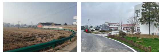
Comparison of Road Repair Before and After
